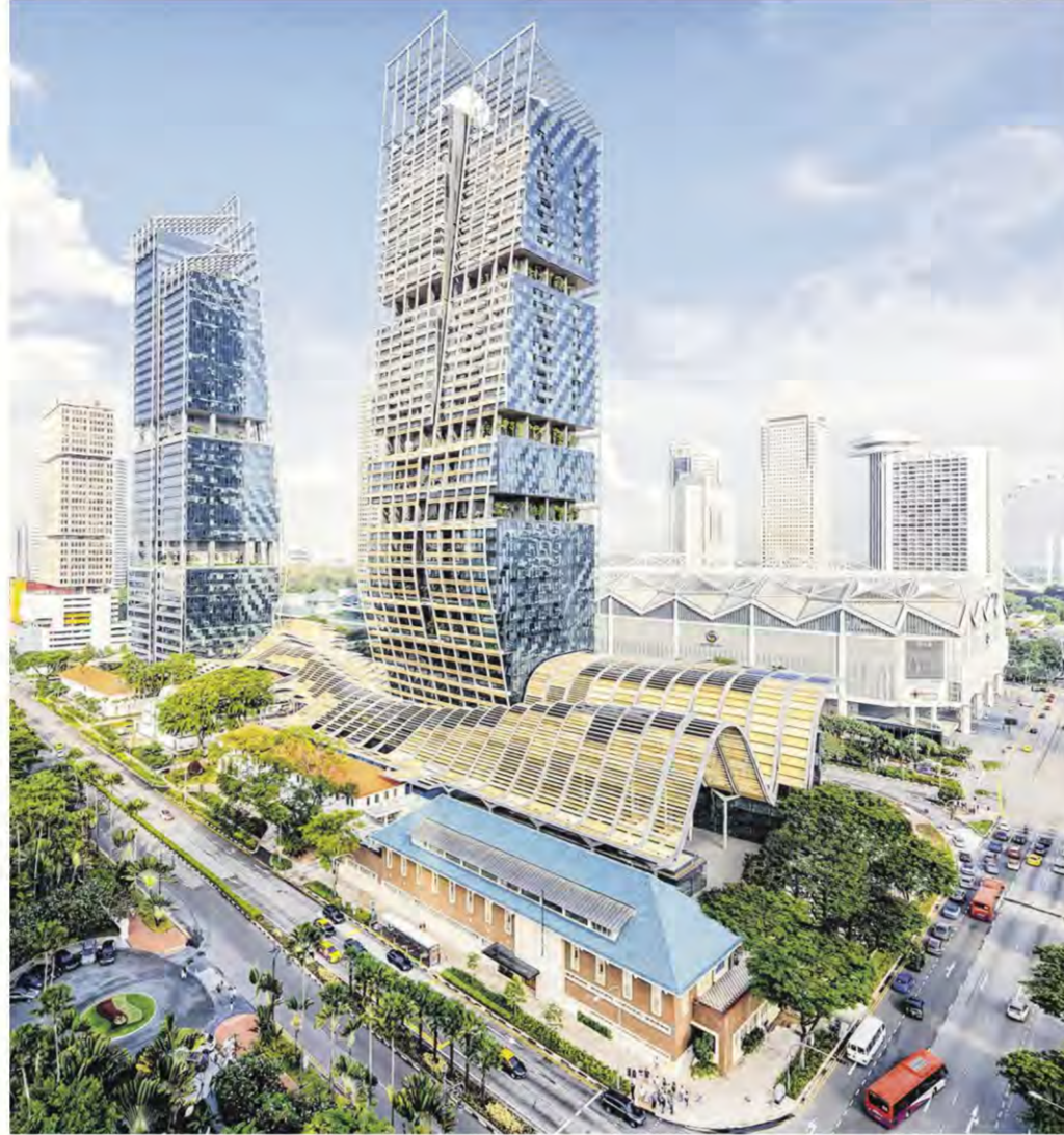
South Beach, CDL's joint venture mega mixed-use development on Beach Road, is a sustainable development with its distinctive microclimatic wave-like canopy which acts as an environmental filter.
